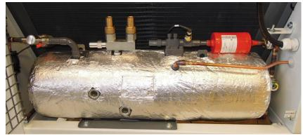
Figure 20: Liquid receiver with safety group
