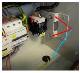
Figure 31 : Main switch position & power supply connection
