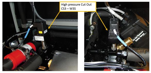
Figure 18: High pressure cut out device
