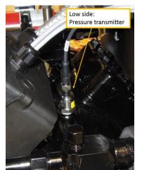
Figure 22: Low side pressure transmitter
